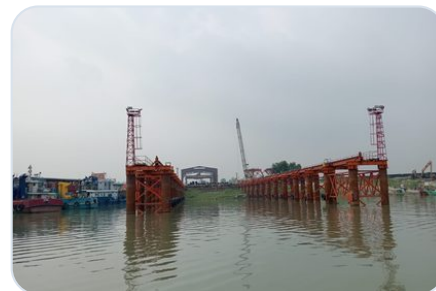
Jetty & steel structure works
