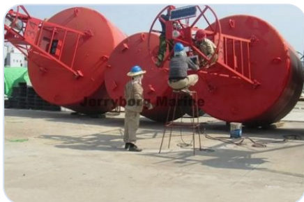
Navigation buoy fabrication & installation
