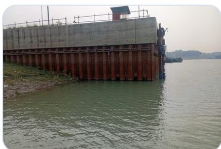
Cofferdam & sheet-pile works
